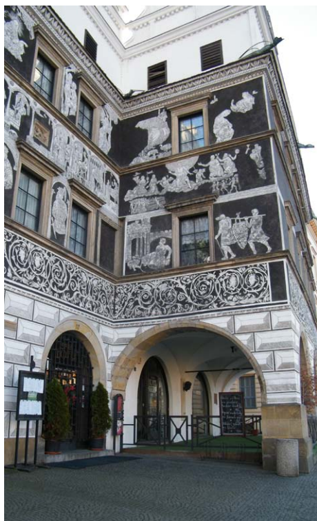
Restaurace a galerie Salva Guarda
